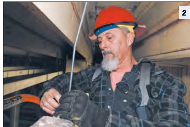
1) Randall Ollenberger, 60th Civil Engineer Squadron electrician, positions an ultra boom lift March 14 at Travis Air Force Base, Calif. An ultra boom lift is a large crane used to lift a person up to reach places in need of repair. 2) Ollenberger lines up hangar door rail March 14 at Travis. Ollenberger had to straighten the hangar door rail so it would work properly. 3) Senior Airman Nathan Kvinnesland, 60th CES electrician, changes an exit sign March 19 at Travis. The 60th CES electricians conducted maintenance inspections on 250 fire alarm systems, which safeguards 27,000 personnel on a daily basis.
